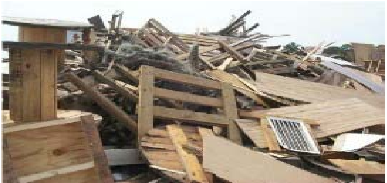
Demolition Debris with Possible CCA Treated Wood
