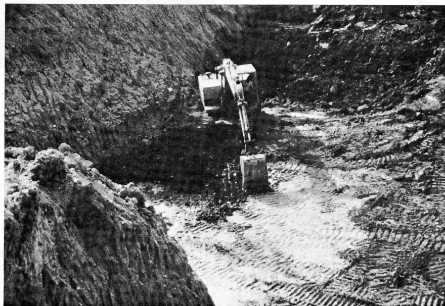
A backhoe struggles against the odds to dig a pit in which drummed wastes will be stored while they wait for a cap of clay.
