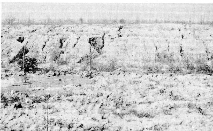
Revegetation over the cap of a hazardous waste disposal pit in Missouri cannot disguise the developing erosion that will plague future generations.
